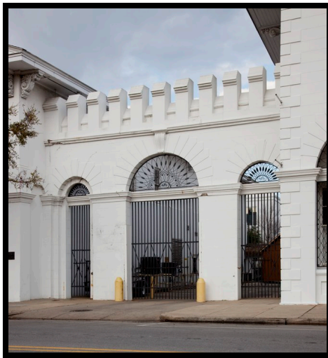
Arches on the Southern Market. Notice the quoins on the building corner also.
